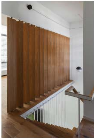
view through angled vertical timber louvers
